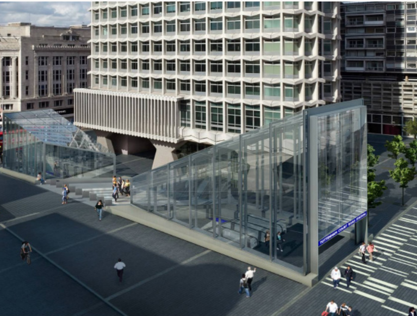
Tottenham Court Road Station
